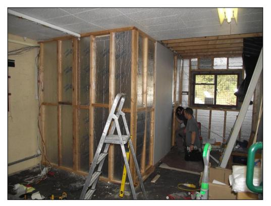
Of course those plans very quickly changed when it was realised that the existing ceiling was supported by the wall and so this was taken down and had to be replaced. Work also got underway on putting in the new timber joists to carry the ceiling. Another skip was on site for all of the rubbish but almost as soon as some of it was thrown in, the "wood magpies" were on hand to saw it all up and take it away for burning; Not a problem as it gave more room in the skip for the general rubbish.
